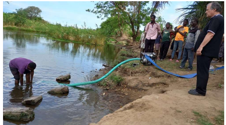
Delivered and now testing one of the water pumps in Chikwawa district
